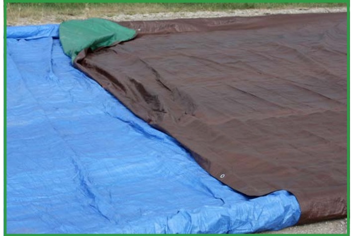
Place uphill tarp over downhill tarp with at least a 6 inch overlap to contain wastewater
