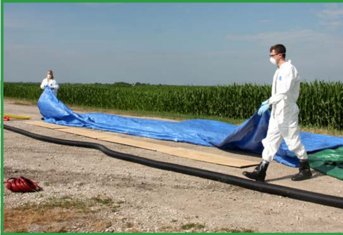
Lay the tarps out over the plywood and berm material
