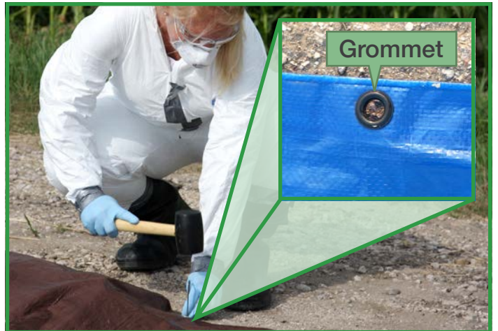
Use stakes to secure the tarp to the ground through the grommets if surface allows
