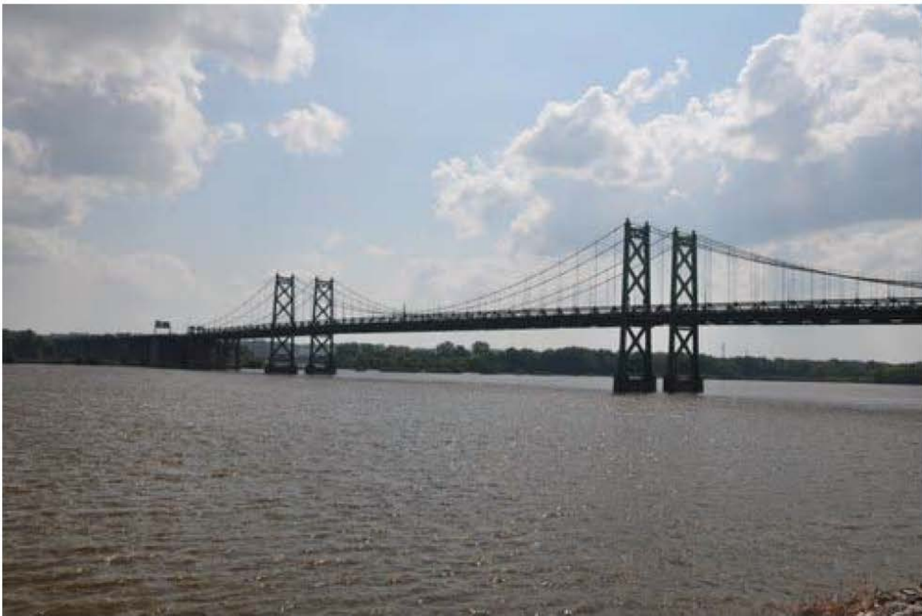
Mississippi River Bridge – Davenport, IA
