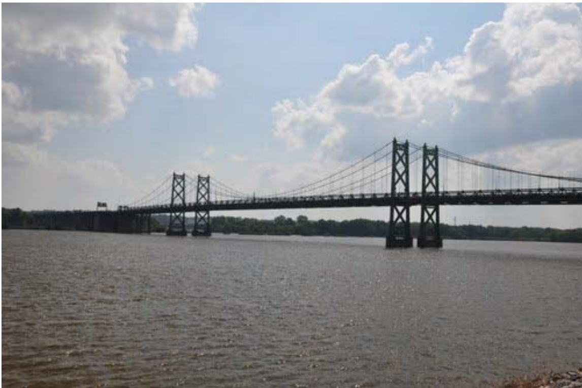
Mississippi River Bridge – Davenport, IA
