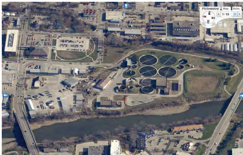
Current view of the North Plant
