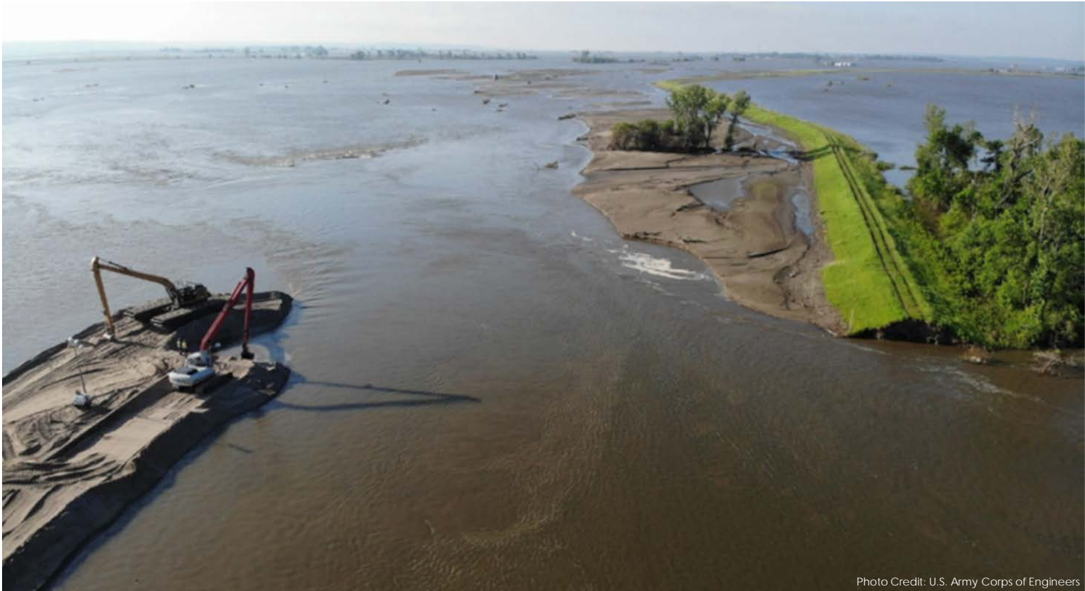
L-575_A_I breach and interim repair, 3 miles north of Percival (June 2019)
